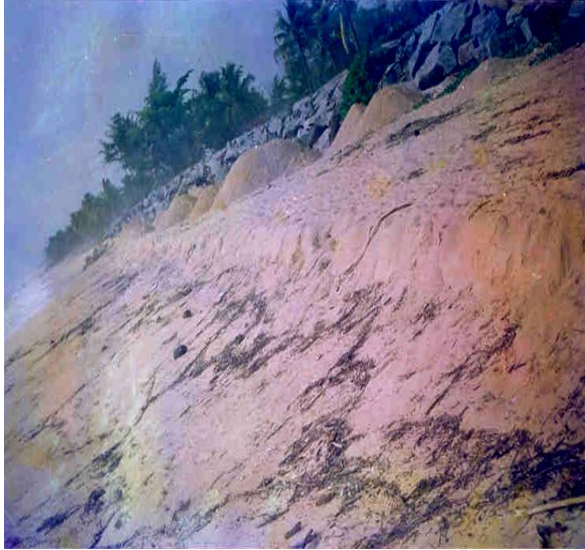
Full stretch of completed seawall
