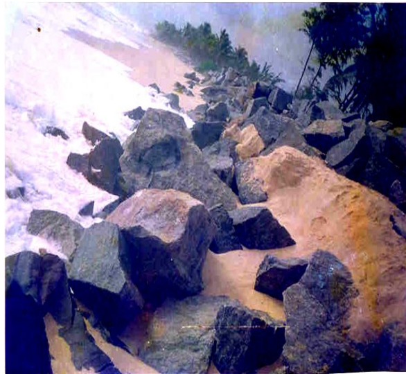
Failure stretch of seawall
